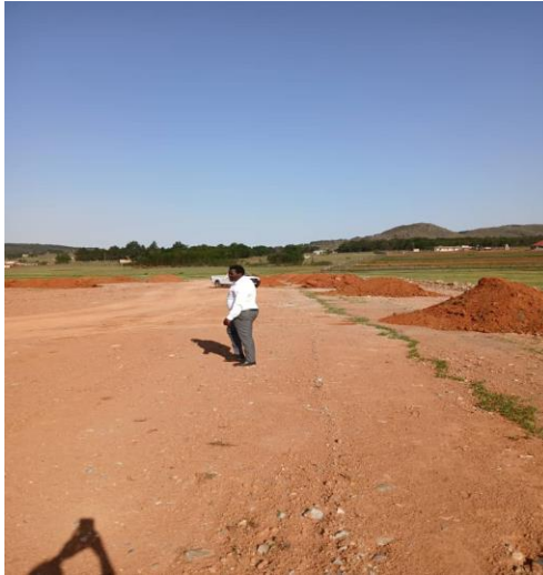
PICTURE 10: SPORTS CENTRE CONSTRUCTION
